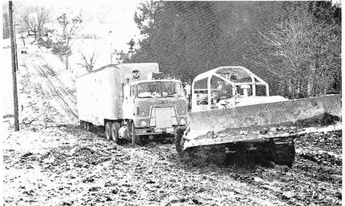
FIG. 6 Even delivering transmitters to some of the sites was a major project, but with the help of a bulldozer the RCA van made the grade.
