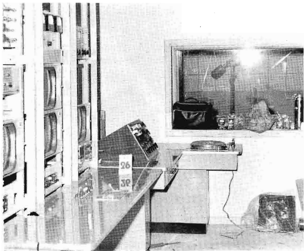
FIG. 8 Terminal and control area looking thru to announce booth.
